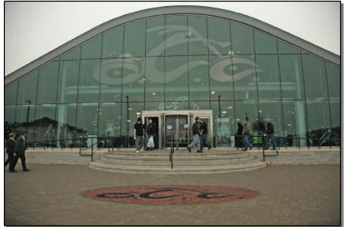
OCC headquarters in Newburgh, N.Y., where the “Impossible Tour” recently visited: OCC chose Grundfos MAGNA variable speed pumps for the facility to circulate fluids in its state-of-the-art radiant heating system.
